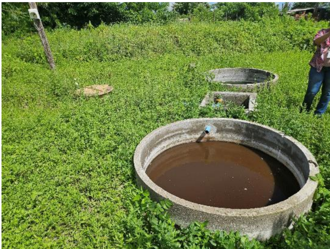
Photo 50 - Gray water reuse system in the São Domingos settlement in the municipality of Cubati
