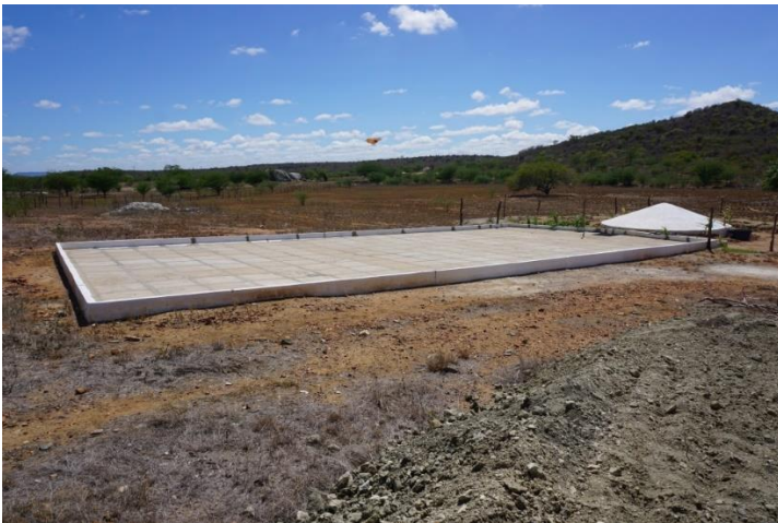
Figure 06 - Rainwater harvesting boardwalk with its 52,000-liter cistern. 112
