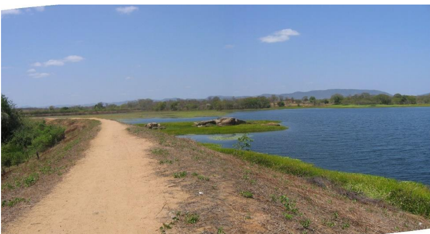
Figure 03 - Weir, seen from the wall or overhang - in the municipality of Cajazeiras, PB 106
