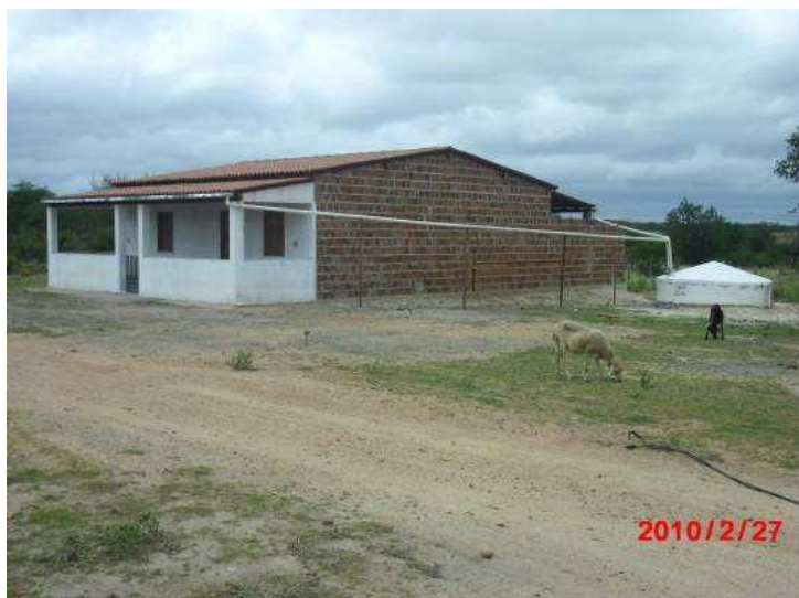
Figure 05 - House with first-water cistern 109
