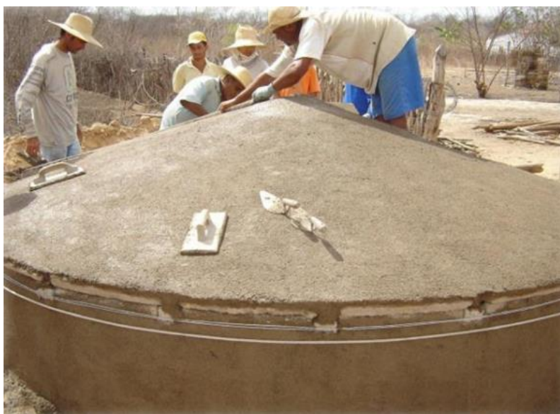
Figure 30 – Cistern construction
