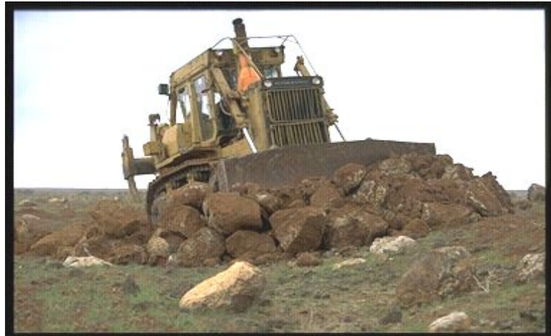
Bulldozers clear fertile land covered with volcanic rock
