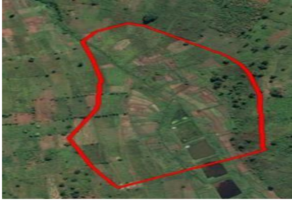
Date: June 2011 Dam in village Kabungwe, Karengwe II, 6 ha
