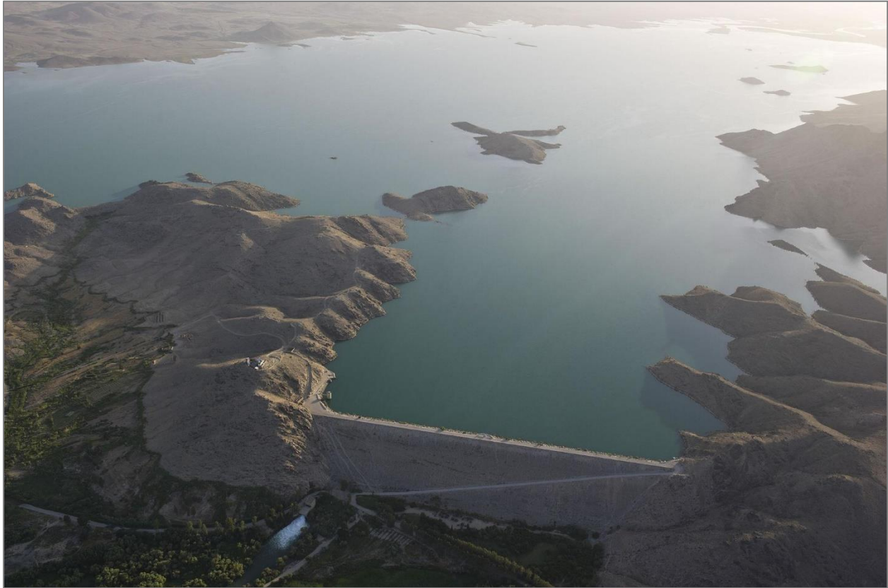
Figure 3. Aerial View of Dahla Dam
