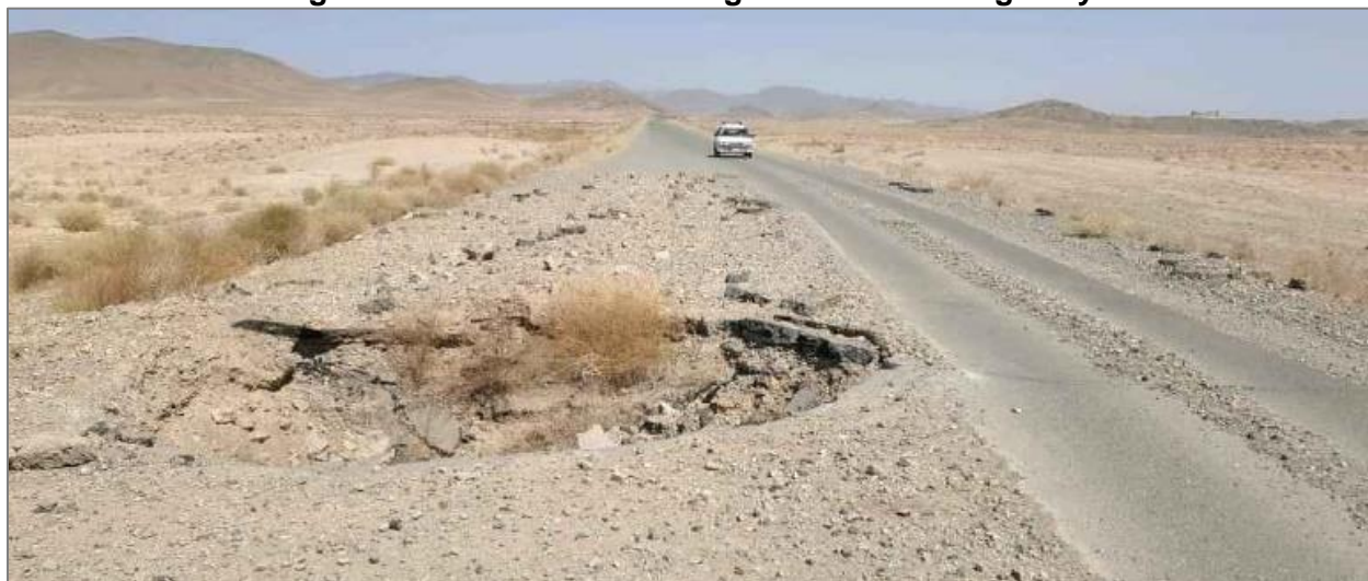
Figure 7. Photo of the Existing Route Bearer Highway
