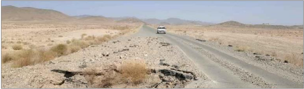
Figure 4. Photo of the Existing Route Bearer Highway
