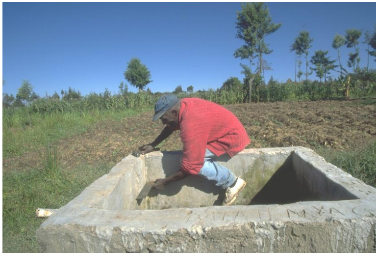
A worker repairs an irrigation chamber Source: Giacomo Pirozzi (IFAD)
