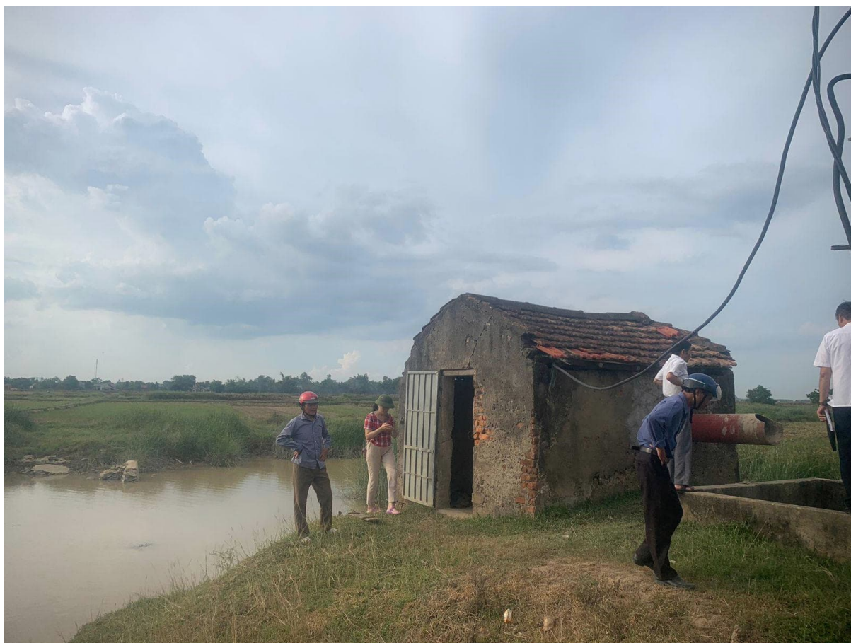
Community managed pumping station identified for upgrade in Chau Nhan commune, Hung Nguyen District, Nghe An
