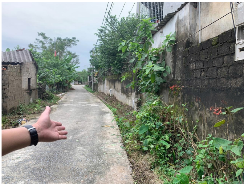
Irrigation canal through residential area
