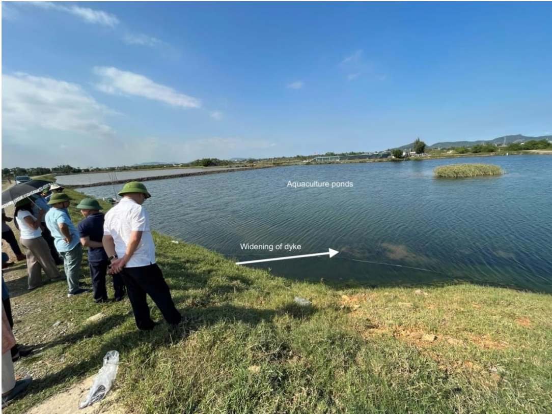
Upgrade of dyke affecting aquaculture activities
